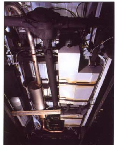
Water tanks are custom made to fit below the floor, which maximizes interior storage space. Locating them between the axles improves weight distribution for better handling.
